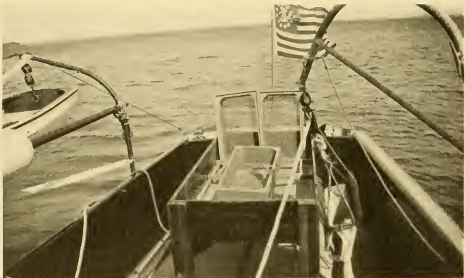
Fig. 15 Rack for sieves, sieves and table. Note strip along which rack slides.
