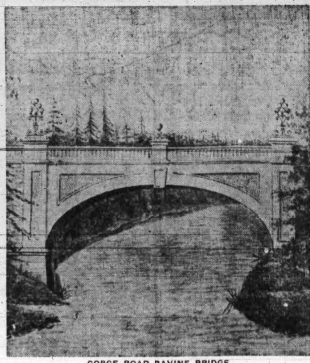
GORGE ROAD RAVINE BRIDGE
