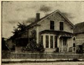
A No. 3015 IDEAL Boiler and 175 ft. of 38-in. AMERICAN Radiators, costing the owner $125, were used to Steam heat this cottage.
