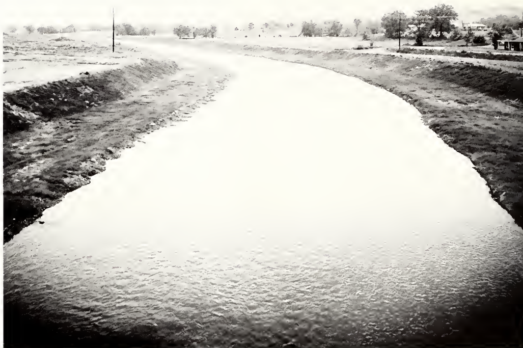
Fig. 4. Widened and relocated channel of West Prong Little Pigeon River, Sevierville, TN, May 1967, looking upstream from U.S. 411 and 441 Highway bridge. McMahan site on left bank beyond bend in the river. Photo courtesy Tennessee Valley Authority.
