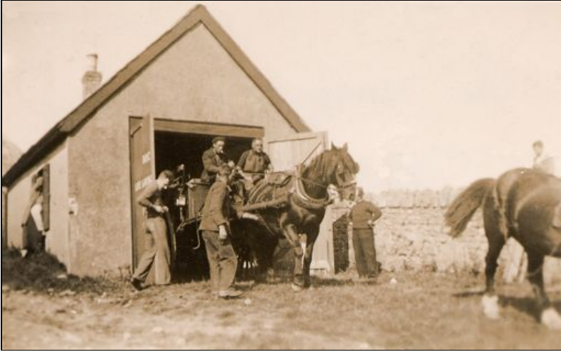
Figure 32: The Rocket Shed in 1922. Photo: The late A.E. Blackwell. Myrtle Ternstrom collection
