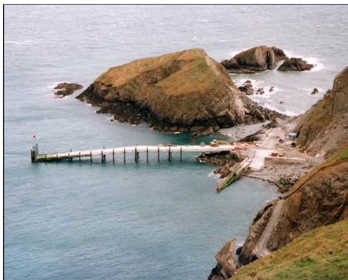
Figure 43: The pier constructed by 1999. The slipway built by Christie is just to the right of it. Photo: M. Ternstrom
