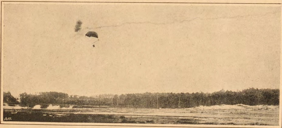
The effect of the "tell-tale" shell, for use with the Krupp Aerial Defence Gun, is indicated in the photograph, which shows the trail of smoke which the projectile leaves behind.
