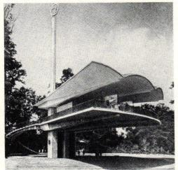
Above: Architektur und Wohnform, No. 6, Stuttgart. The cement industry's building at the 1951 Hanover exhibition is this fanshaped reinforced concrete platform, approached by a curving ramp and covered by a wavy concrete bonnet.
