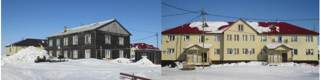
Figure 8.22: Residential houses in Gyda
