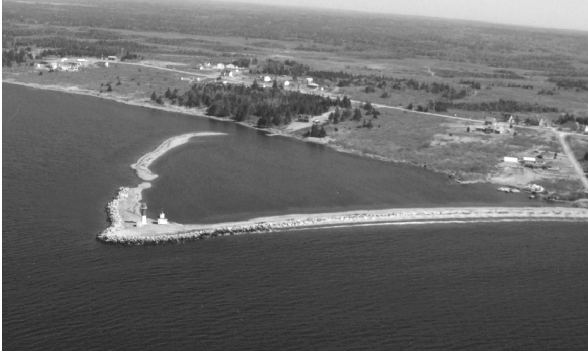
PUBNICO HARBOUR AT BEACH POINT (2000)
