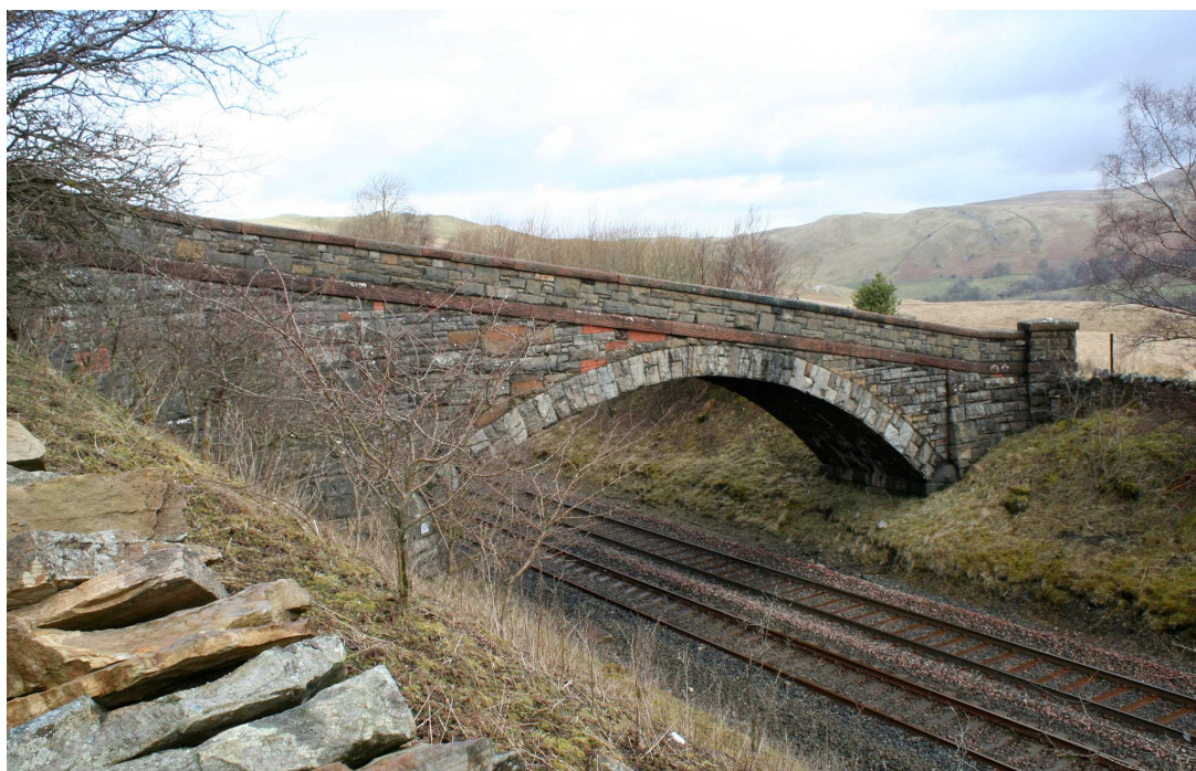
Plate 9: Bridge 14 crossing the railway
