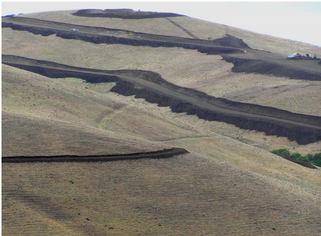
Figure 29. Access roads being prepared for wind turbines in Klickitat County.
