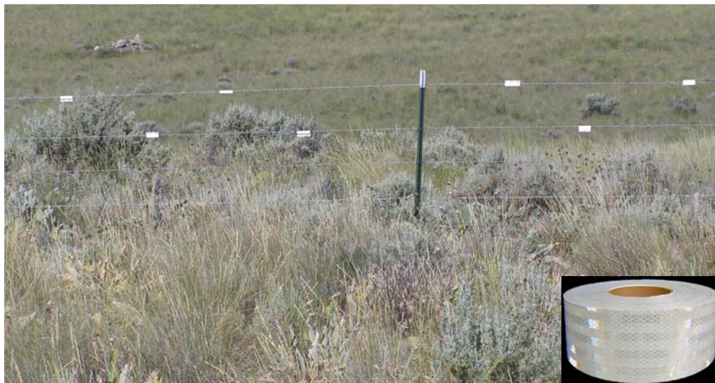
Figure 32. Fence near West Foster Creek marked with vinyl markers, and (inset) heavy duty reflective tape to use on smooth wire.
