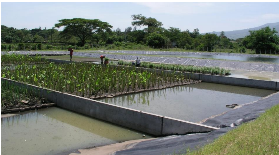
Figura 7: Constructed wetland ( "Constructed Wetlands," 2015)
