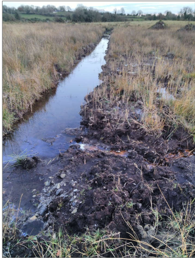
Recently installed drain
