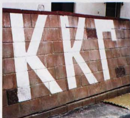
Wall cracks and other structural damage are prevalent at the Epsilon Xi house.
