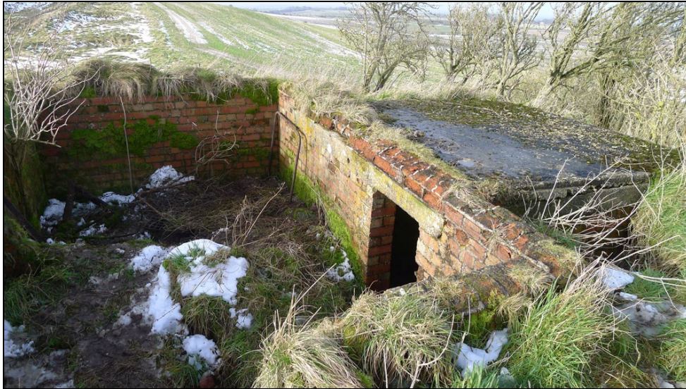
Fig. 6 Gun pit with rear blast shelter
