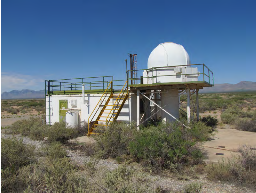
Figure 32. Type "B-SS" Instrumentation Stand, NW 50 Site, WSMR.
