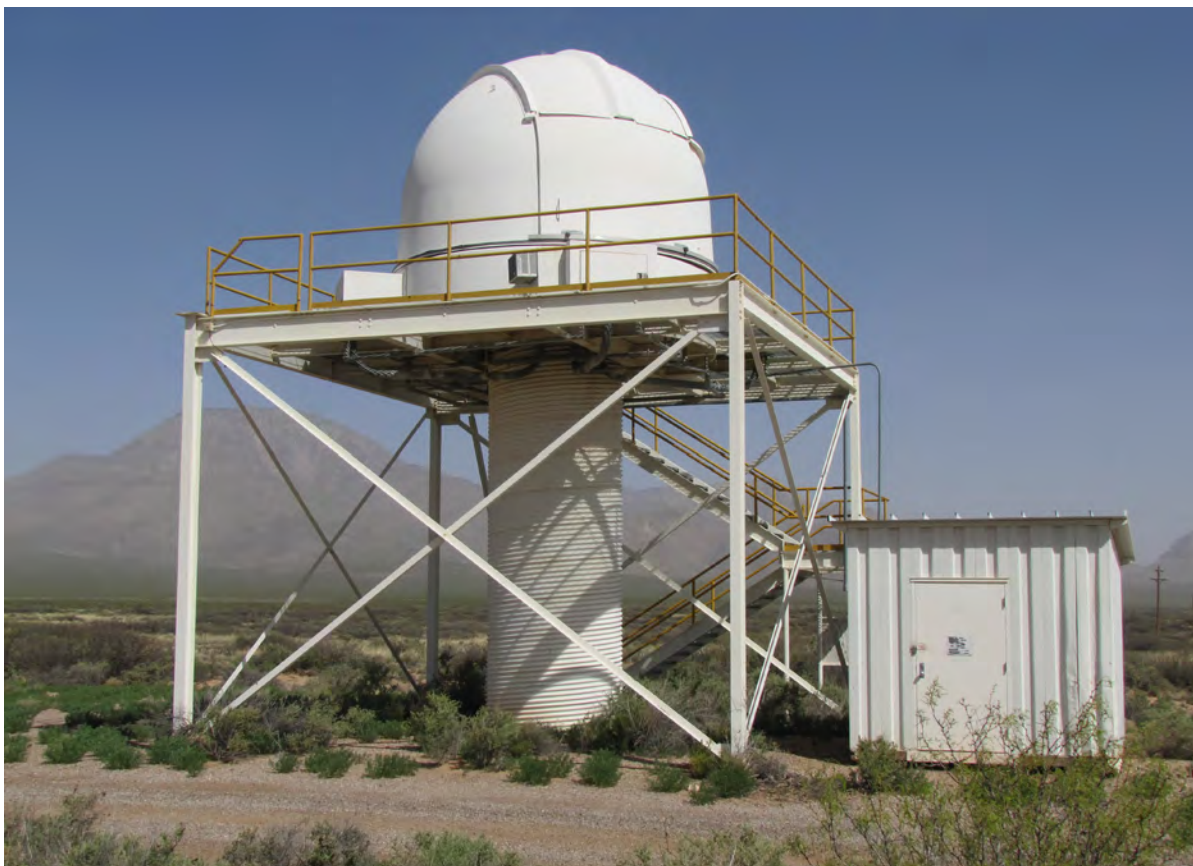
Figure 42. 20-foot fixed telescope stand with 16-foot Tommy Tower Astrodome, NW 50 Site, WSMR.
