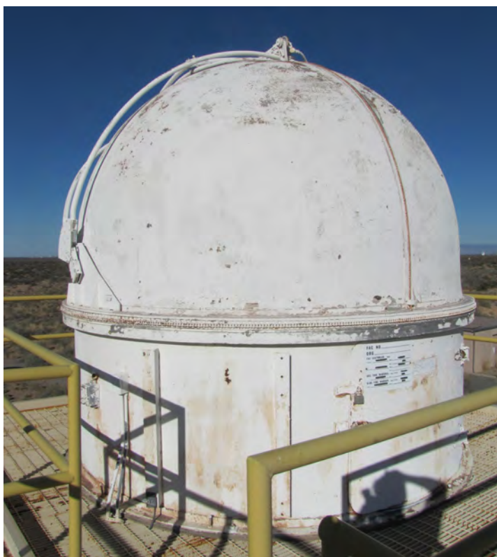
Figure 20. Houston Fearless fixed astrodome at the former HIDL, White Sands Missile Range.
