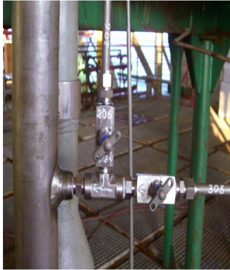
FIG. 19. Separator sampler used for water sampling in oil wells.
