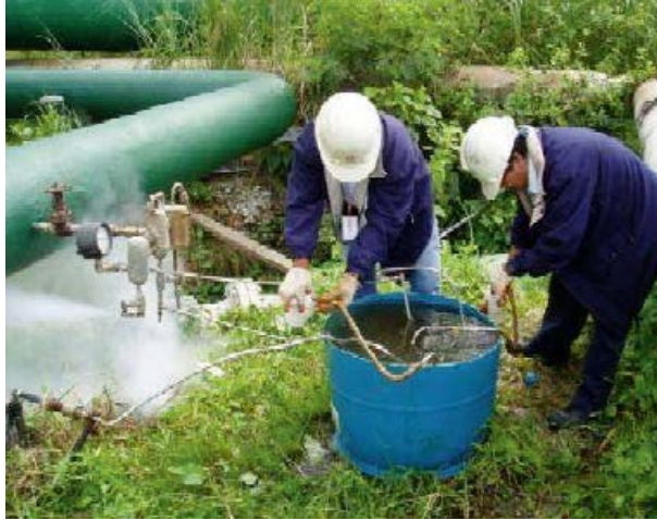
FIG. 16. Sampling of HTO in a geothermal well in the Philippines using a Weber separator.
