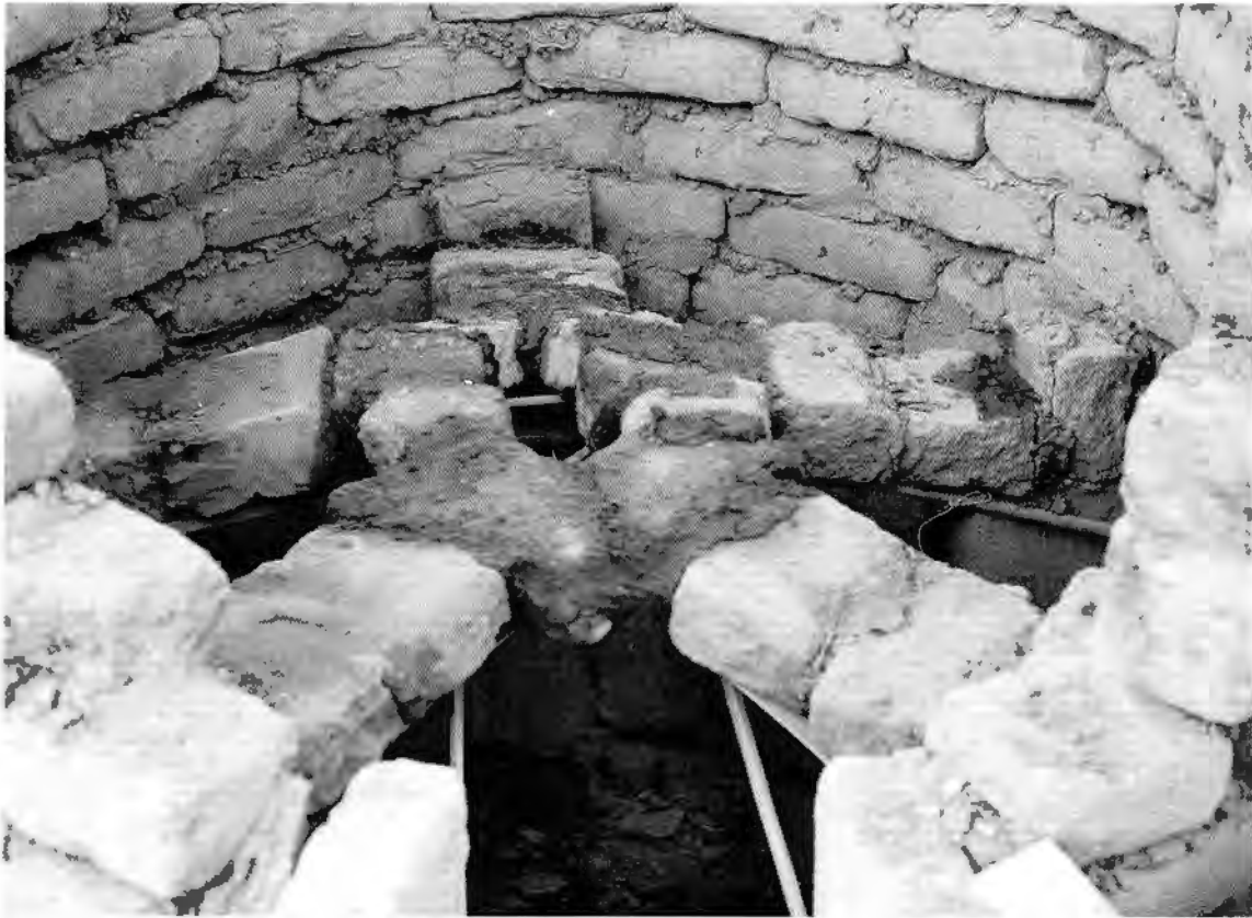
Figure 8.9. The completed fenestrated dome before plastering and burning out the former.
