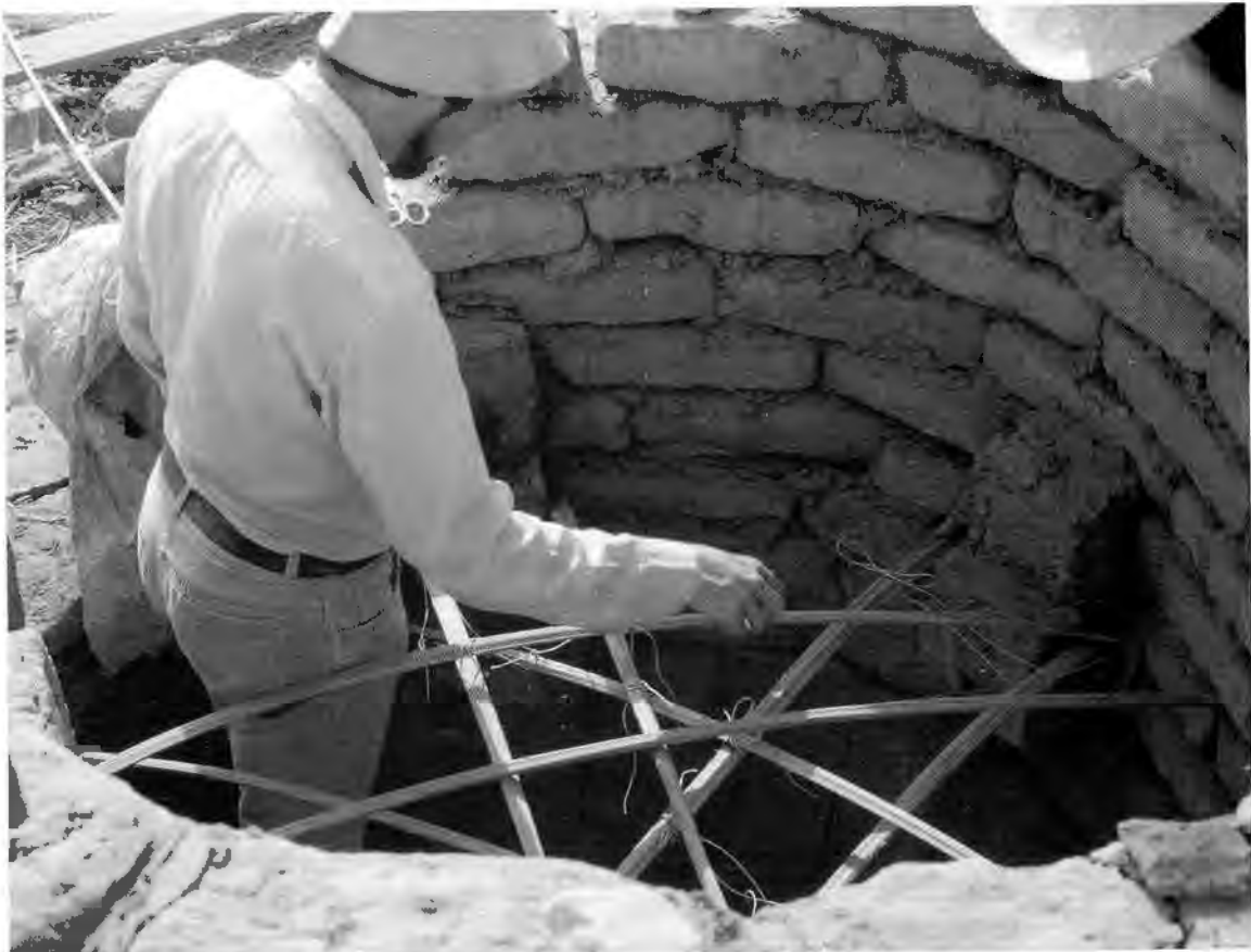
Figure 8.8. Making the gereed former for the fenestrated dome of the kiln floor.
