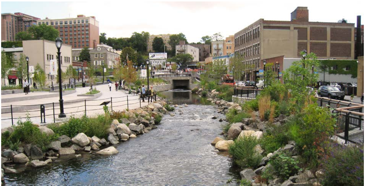
Saw Mill River after completion of daylighting, Yonkers, NY | Groundwork Hudson Valley
