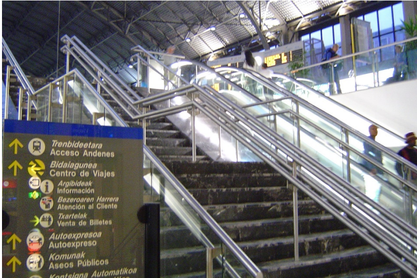
Handrails at varying heights to accommodate users San Sebastian Central, Spain
