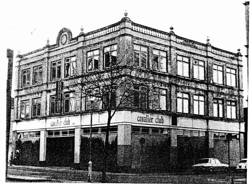
FIG. 6. Jarrow & Hebburn Co-operative Society Ltd, Drapery Depot, Jarrow (1904). Hennebique system. Architect: J. Cordiner. (Photographed 1977).
