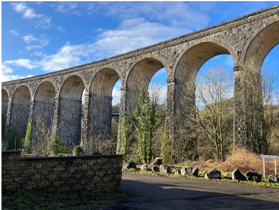
Figure 6 Cefn Railway Viaduct
