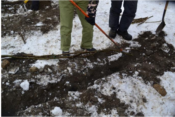
Figure 5. Digging a trench for fascine installation. Photo by AWES.
