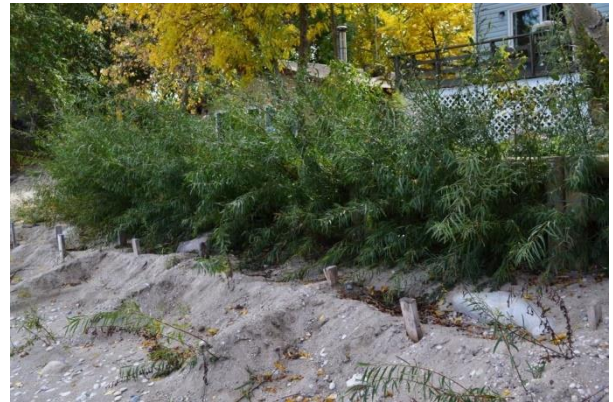
Figure 6. A fully grown fascine of sandbar willow ( Salix exigua ). Photo by AWES.
