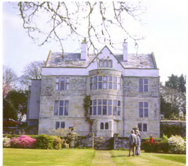
Tremeer, a Cornish 14th Century country house constructed of local granite, has weathered well across the centuries. Running along the base of the terrace is a large collection of Kurumes from Yokohama Nurseries that was introduced by John B. Stevenson (seen in April 2002).
