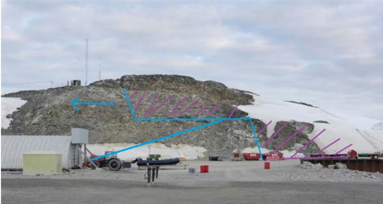
Figure 6 – Quarry stage 2 showing the upper face progression towards the north.
