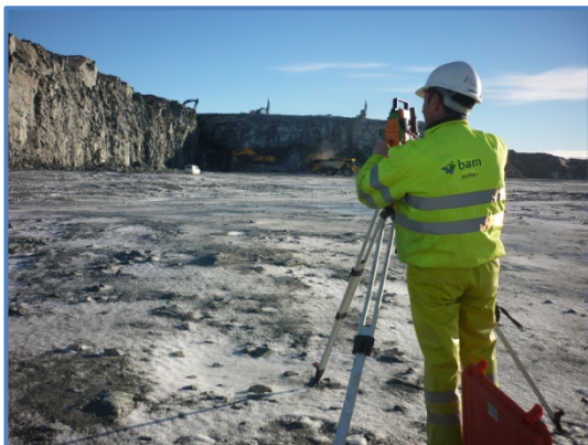
Figure 29 – Undertaking a laser profiling survey of the face
