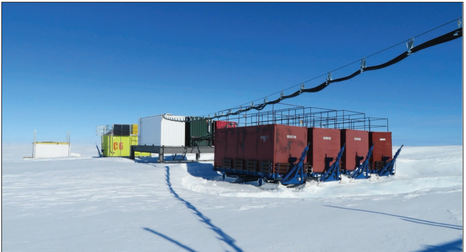
▲ The Automation Platform with four bulk fuel tanks that the containerised microturbine system autonomously fuels from throughout the unmanned winter. We did not raise any infrastructure at Halley in 2020/21 due to the small team and short time available to us, so we're expecting the infrastructure to be a little more buried than usual
