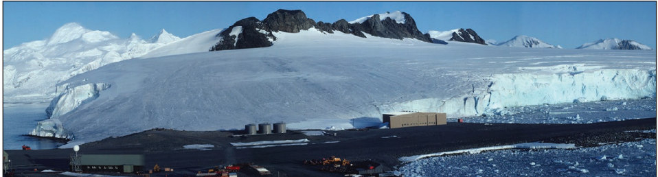
▲ The ramp at Rothera Research Station in early 1992
