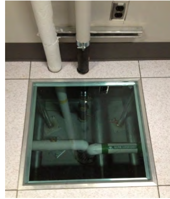
Figure 2: Raised floor
