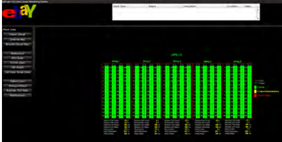
Figure 19: Server rack aisle power monitoring
