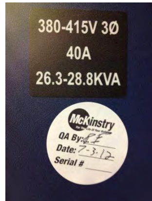
Figure 18: QA procedure verification and sign-off by team member
