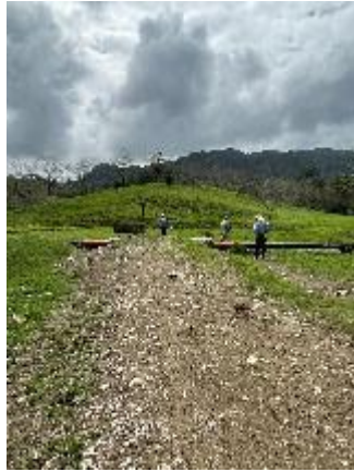
Photograph 19 Aqueduct of the Guitarras estate.
