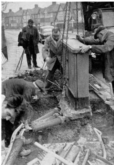
MOVING THE CABINET WITH THE HELP OF A JUMBO CRANE
