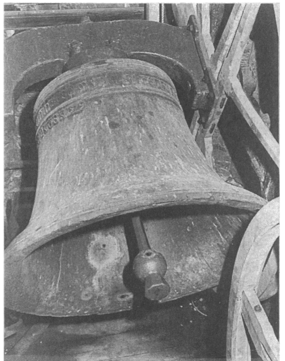
FIG 4—Swinging bell with clapper bolt protruding from top of headstock. This bell weighs 579 kg (fifth bell, Sutton Bonnington)
