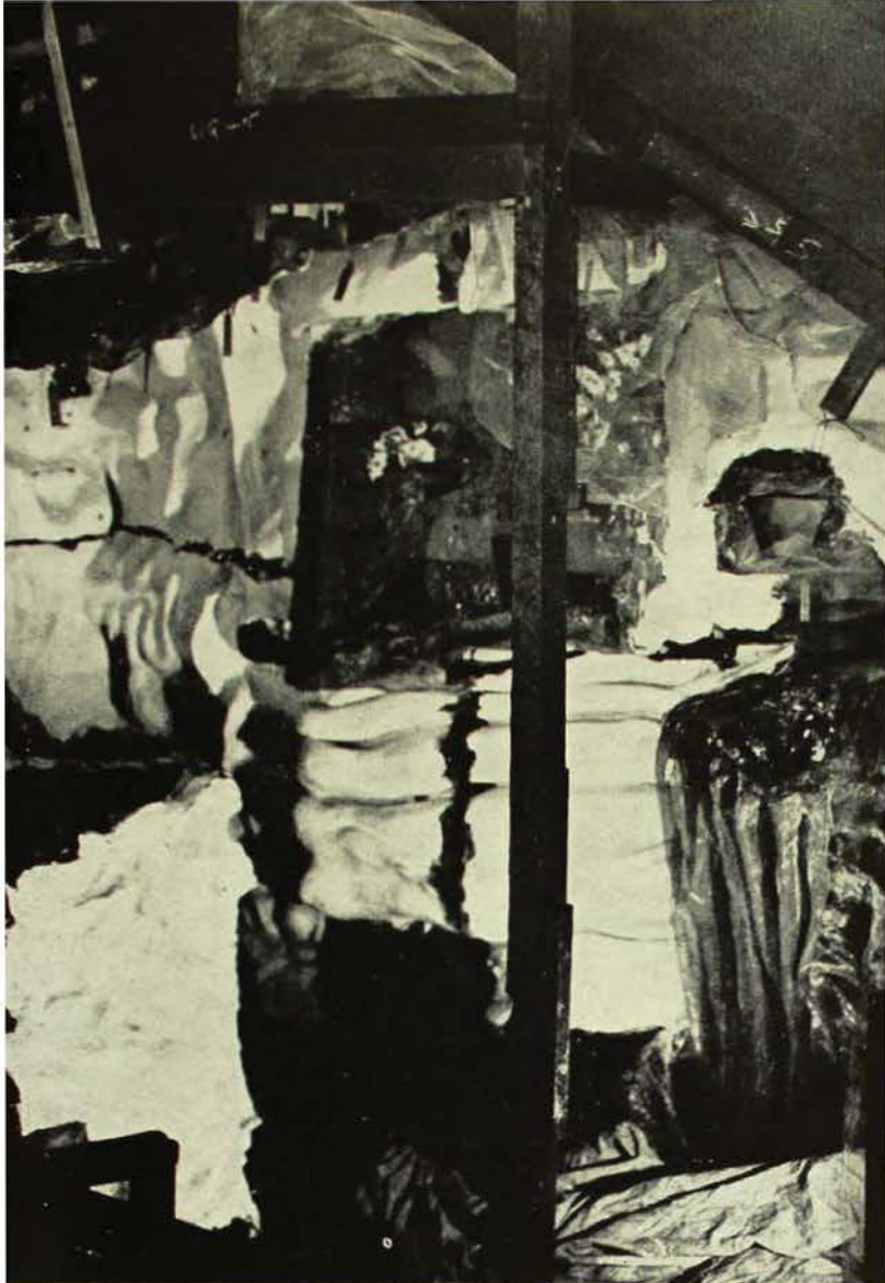
A further stage in the construction; the gauze is here seen in process of being covered with the composition used in making the rock. In the bottom left hand corner is the rock upon which the broken column is to rest.
