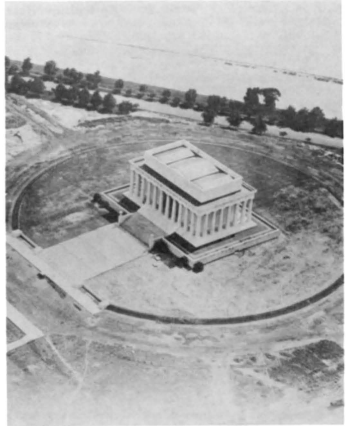
The beginning on reclaimed land.
