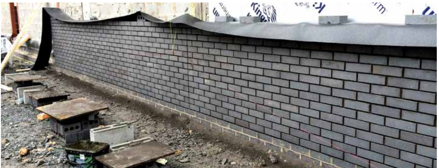
Protection from rainfall, note stacks of bricks also covered
