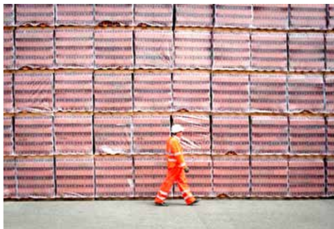
Stored bricks must be protected from inclement weather.
