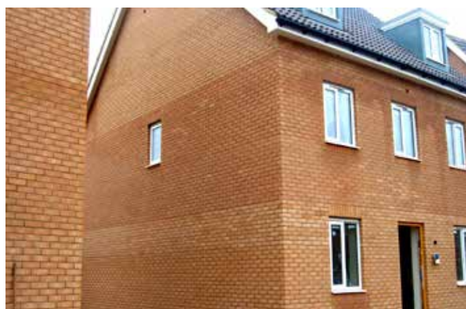
Poor blending of bricks can result in unsightly banding or demarcation lines.
