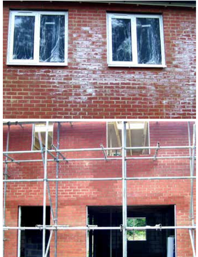
Saturation and efflorescence from unprotected openings.
