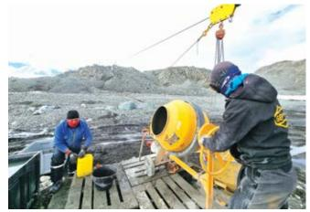
An aerial ropeway carries up a hill cement for the groundwork of the new lab
