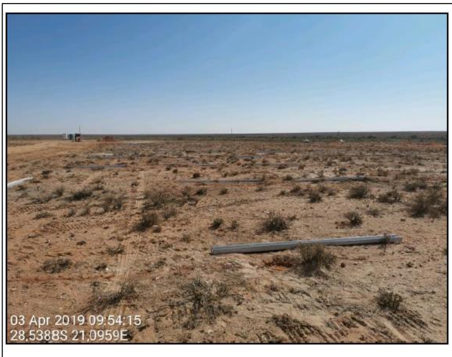
Figure 7: pre-drilled holes are backfilled with a wet sand mixture and steel piles placed in position ready for ramming.
