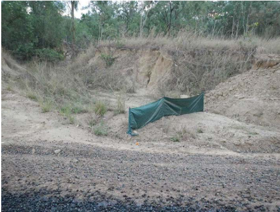
Figure 75 A inadequate silt fence for erosion control that did not follow BMP guidelines (Wetheridge 2009; 2012), was not embedded into gully banks, and is being overwhelmed by road sediment due to overzealous clearing and improperly designed road drainage.
