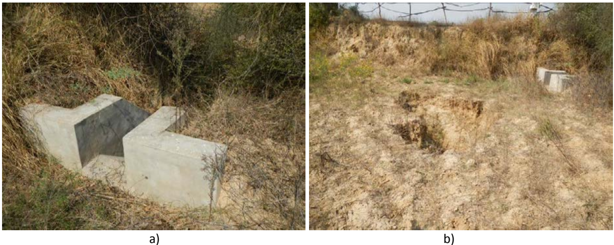
Figure 71 a) A prefabricated drop structure ( sensu Yadav and Bhushan 1994) placed at an alluvial gully headcut in India, and b) water bypassing of the drop structure due to piping and tunnel erosion through the dispersive alluvial soils upslope.
