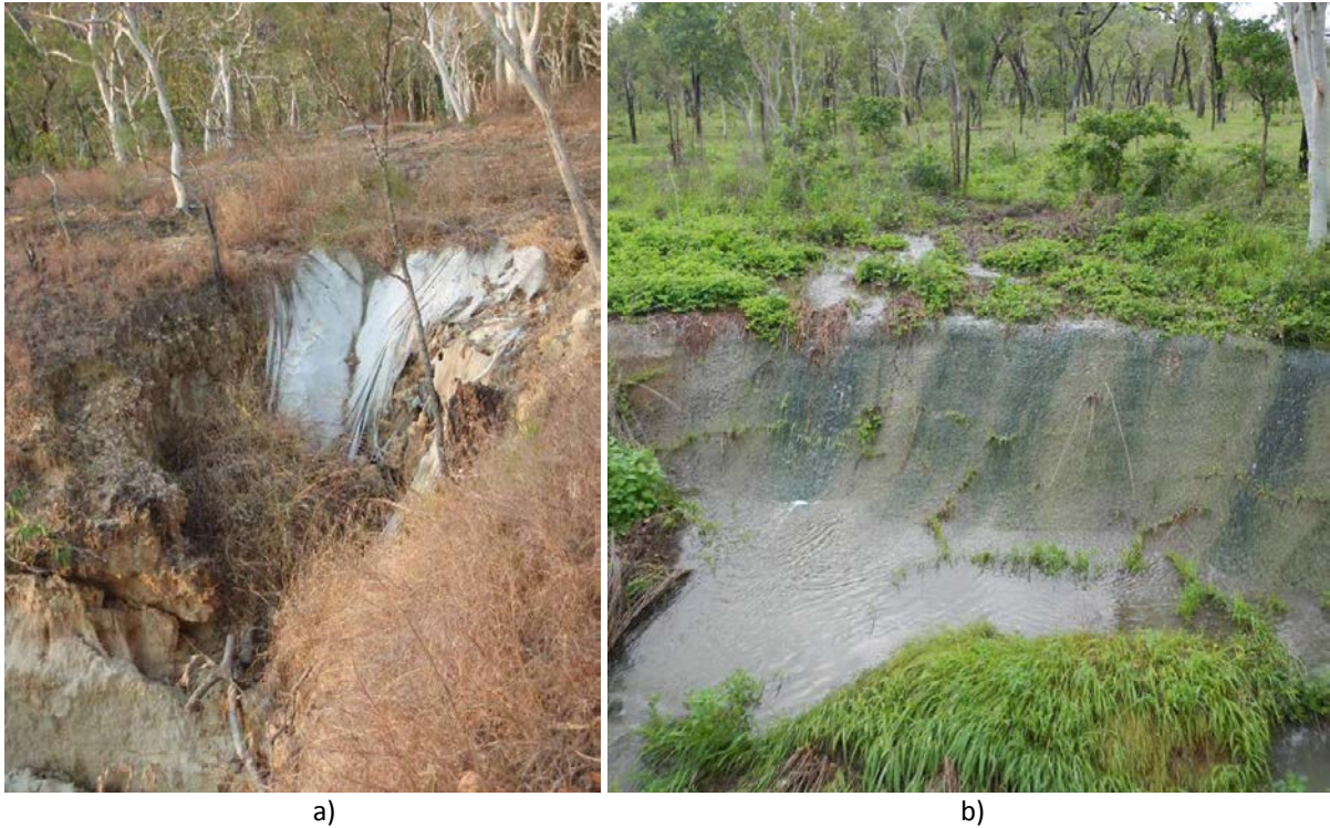
Figure 70 Drop structure examples in the Normanby catchment using a) geo-textile blankets installed at a gully headcut in a failed attempt to protect the soil surface and funnel overland runoff over the headcut, and b) a concrete drop structure and stilling basin at a gully headcut upstream of a road culvert.
