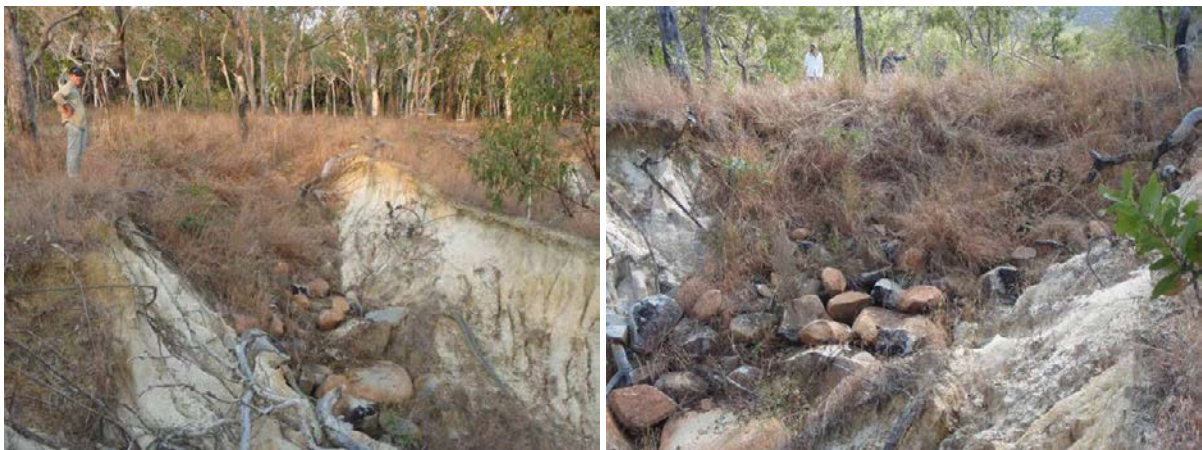
Figure 67 Angular rock armouring and soil backfill at a gully headcut. Note good kangaroo grass ( Themeda triandra ) and black spear grass ( Heteropogon contortus ) establishment on the soil backfill.
