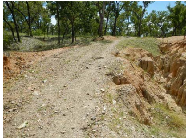
f) After Treatment, After Wet (April-2012)
