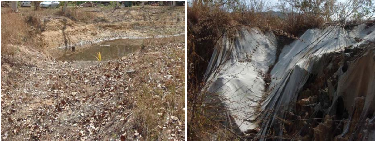
Figure 86 Example of a) a small farm dam installed above a gully head to retain and dissipate overland runoff before reaching the gully head, and b) the gully headcut below the dam still eroding from excess storm runoff out of the dam and insufficient armouring of the headcut.
