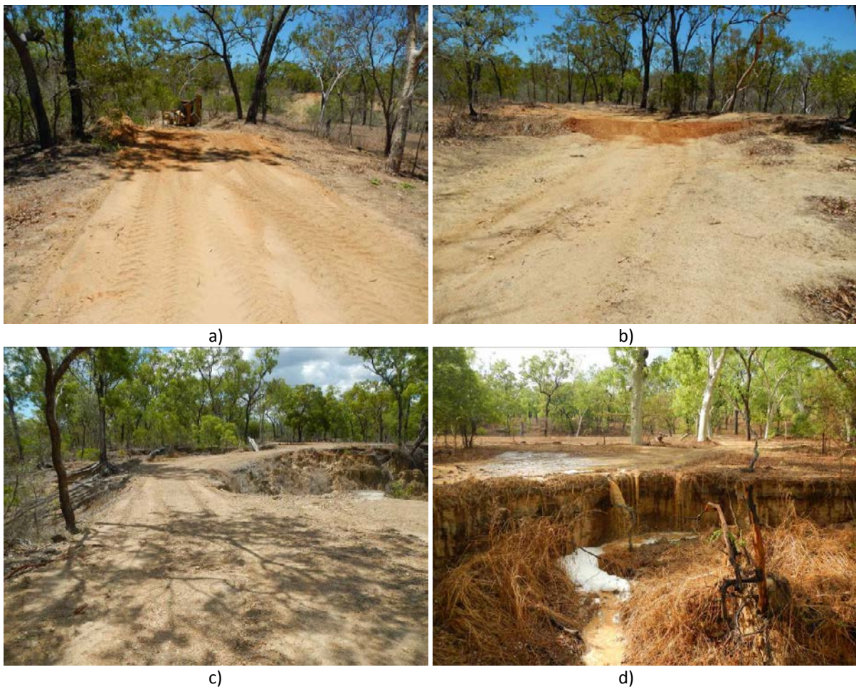
Figure 134 Examples of road improvements along the Granite Normanby road including a) a water diversion bank at the top of a creek approach, RG28 , b) a diversion bank along a long road fetch, RG29, c) gravel sheeting over a narrow road choke point (RG36) to protect the underlying sodic soils from wash and reduce ponding and piping, d) a water diversion bank (in background) used to divert some (1/3) but not all of the runoff water away from this road headcut, RG32.
