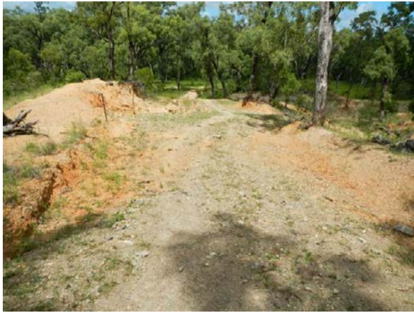
e) After Treatment, After Wet (April-2012)
