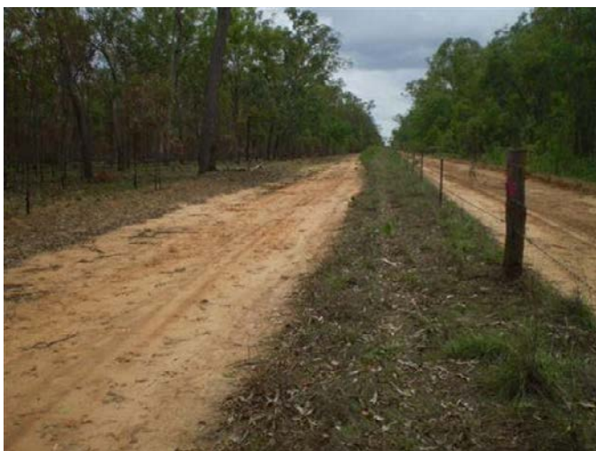
Figure 147 Fence line grading for fire breaks can concentrate water runoff from deep grading and accelerate gully erosion, especially if frequent water diversion banks (whoa boys) are not installed to maintain natural flow paths and mitigate erosion.
