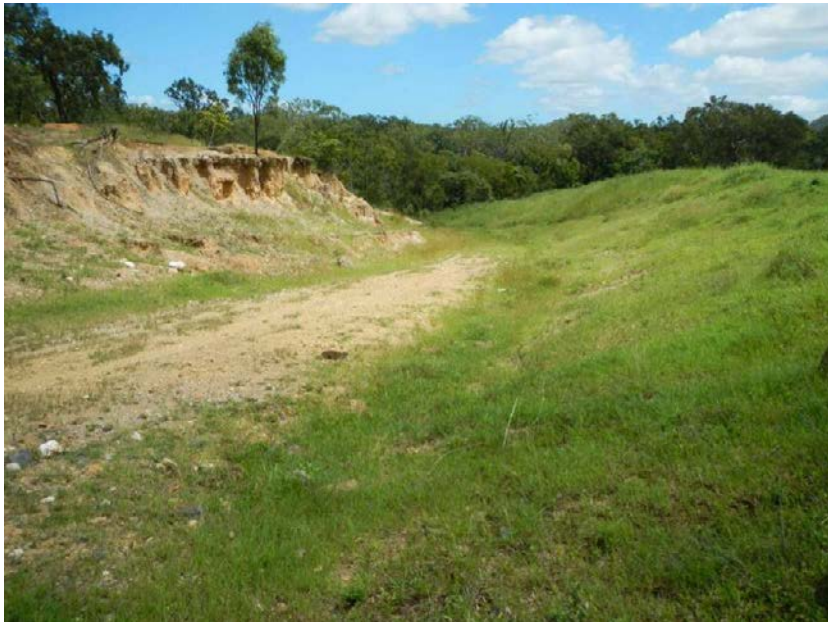
Figure 94 Comparison between the left and right approaches to the south side of the old West Normanby bridge crossing, April 2012. The right side was battered back and revegetated during the decommissioning of the road crossing circa 2006. Note that significant erosion continues down the centre of the old road due to excess water runoff.
