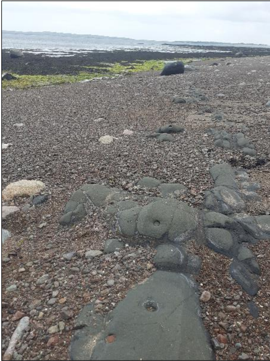
Figure 10: Boreholes in the Dike at Tong - general
