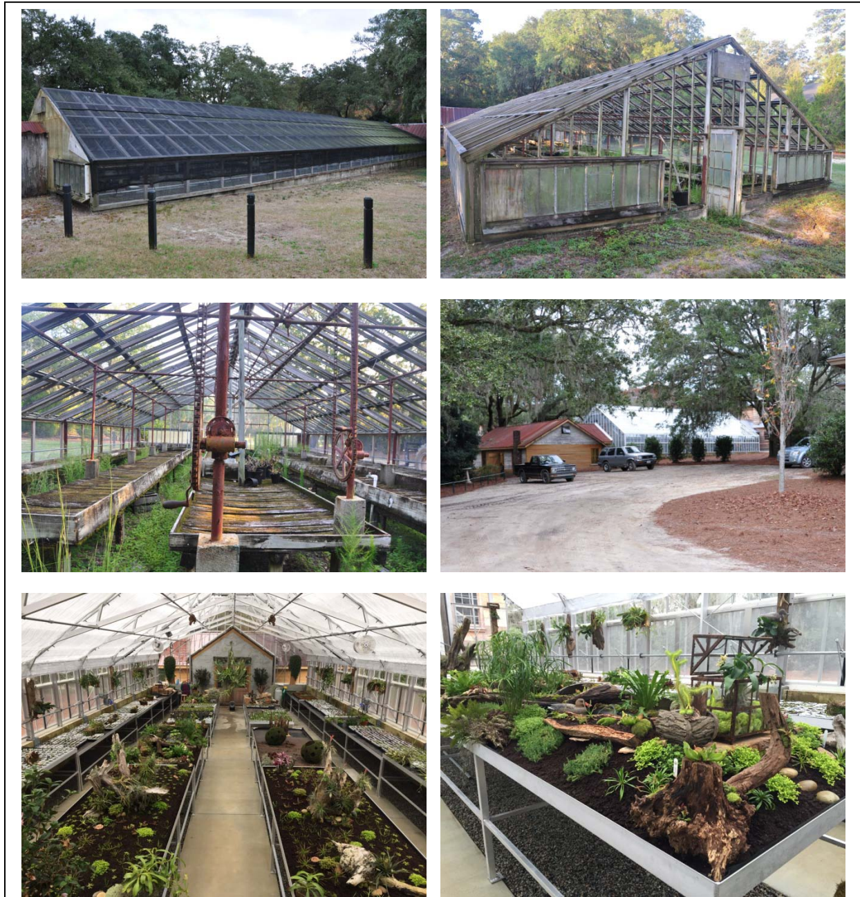
Figure 36. Greenhouse 1. Upper photos show the greenhouse prior to renovations looking southeast and south-southwest. Middle left photo shows the interior prior to renovation. Compare to Figures 22 and 30. Middle right photo shows the exterior after renovation, looking to the northwest. Lower photos show the renovated interior with many of local carnivorous plants.
