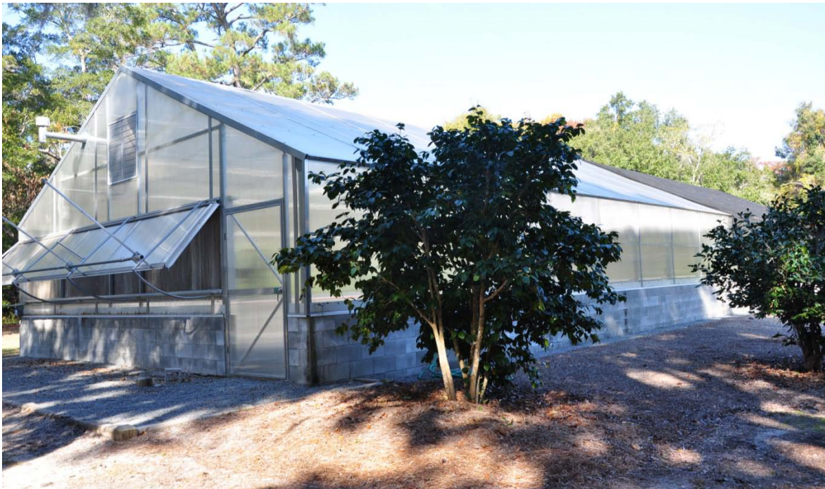
Figure 37. Other Orton greenhouses. Top photo shows Greenhouse 2, looking to the south. Bottom photo shows Greenhouse 3, looking to the southeast. Both greenhouses have been removed.
