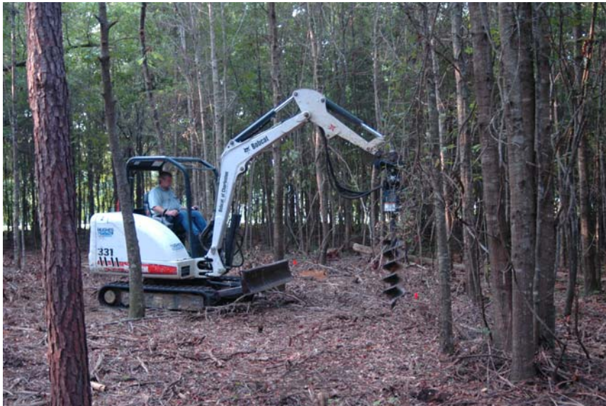
Figure 23. Using a Bobcat to auger at 38CH1693.
