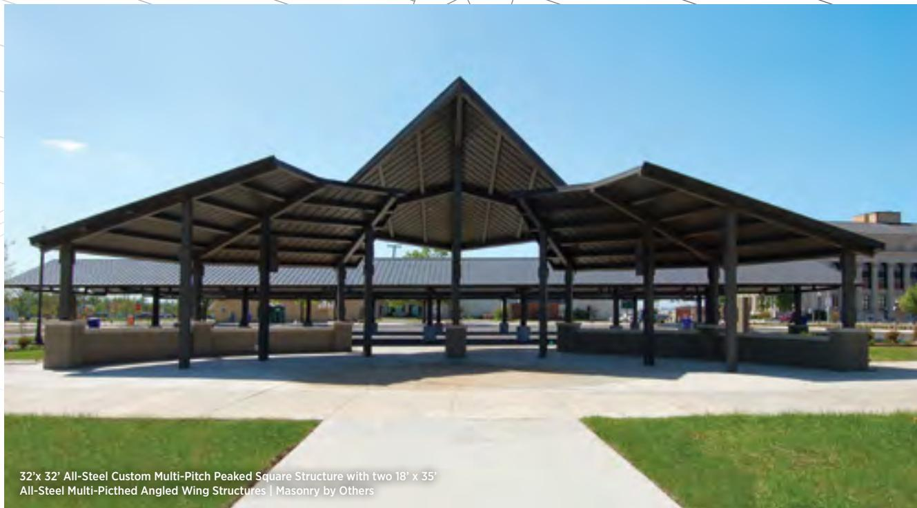
32'x 32' All-Steel Custom Multi-Pitch Peaked Square Structure with two 18' x 35' All-Steel Multi-Pitched Angled Wing Structures | Masonry by Others
