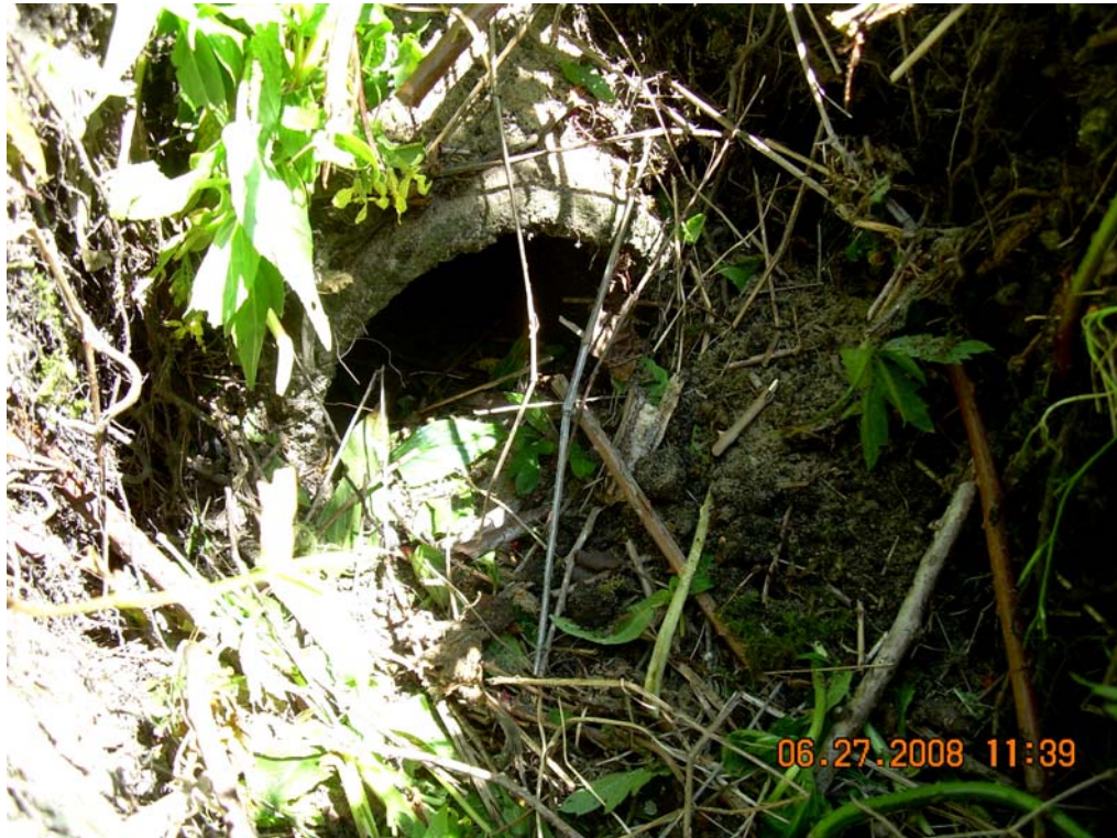
PHOTO 9: Existing stormwater pipe outfall.
