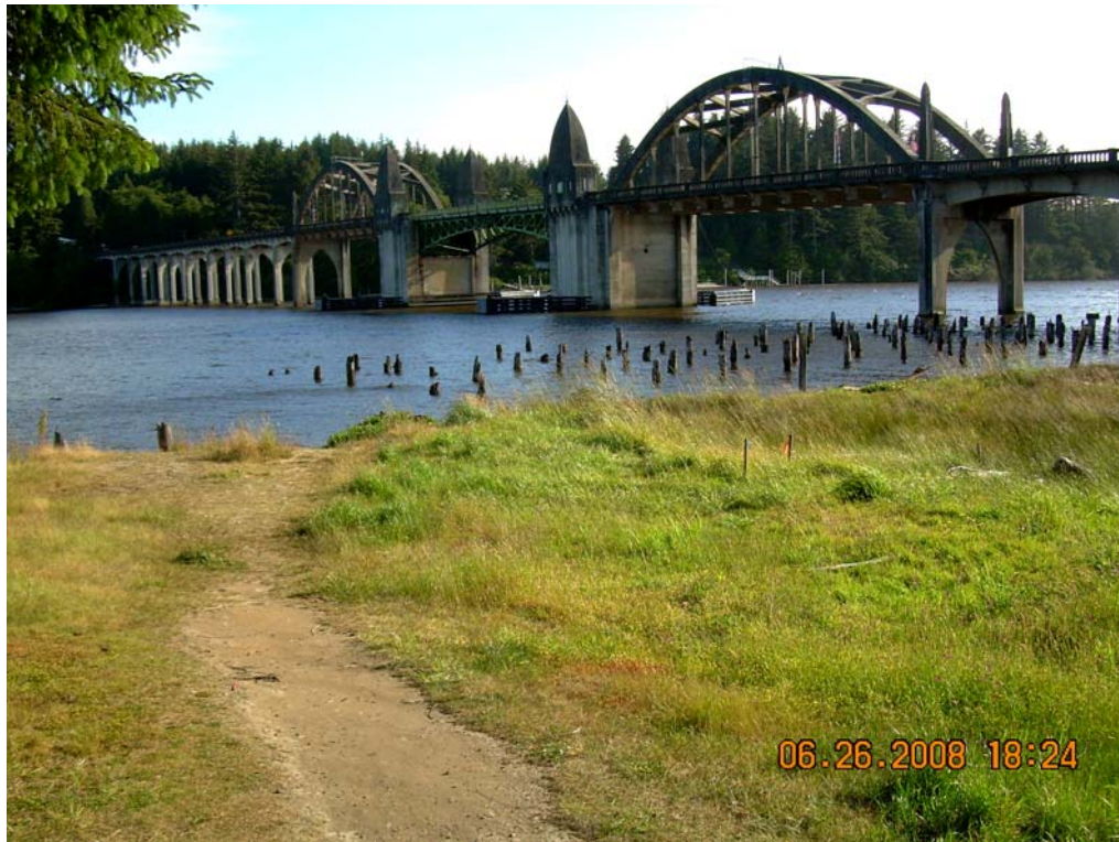
PHOTO 1: Facing south across the project area along the east side at high tide. Existing path is approximate location of the proposed walkway.
