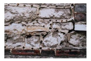
Fig. 6 The picture on the left illustrates how a repair should not be executed. The mortar appears to be applied without any regard for the form of the blocks of masonry, bears no relationship to the original and is already failing.
