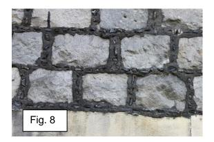
The masonry at Windsor Castle is galleted throughout although very little of it is original. Fig. 7 illustrates some galleting from the time of Henry VIII; earlier galleting is to be found elsewhere in the castle. These provide a useful guide to the correct treatment of masonry for a given period when carrying out repair work.
