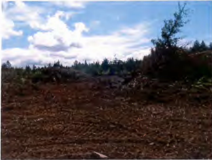
1. April 22, 2016, area that was scrub/shrub has been cleared.
