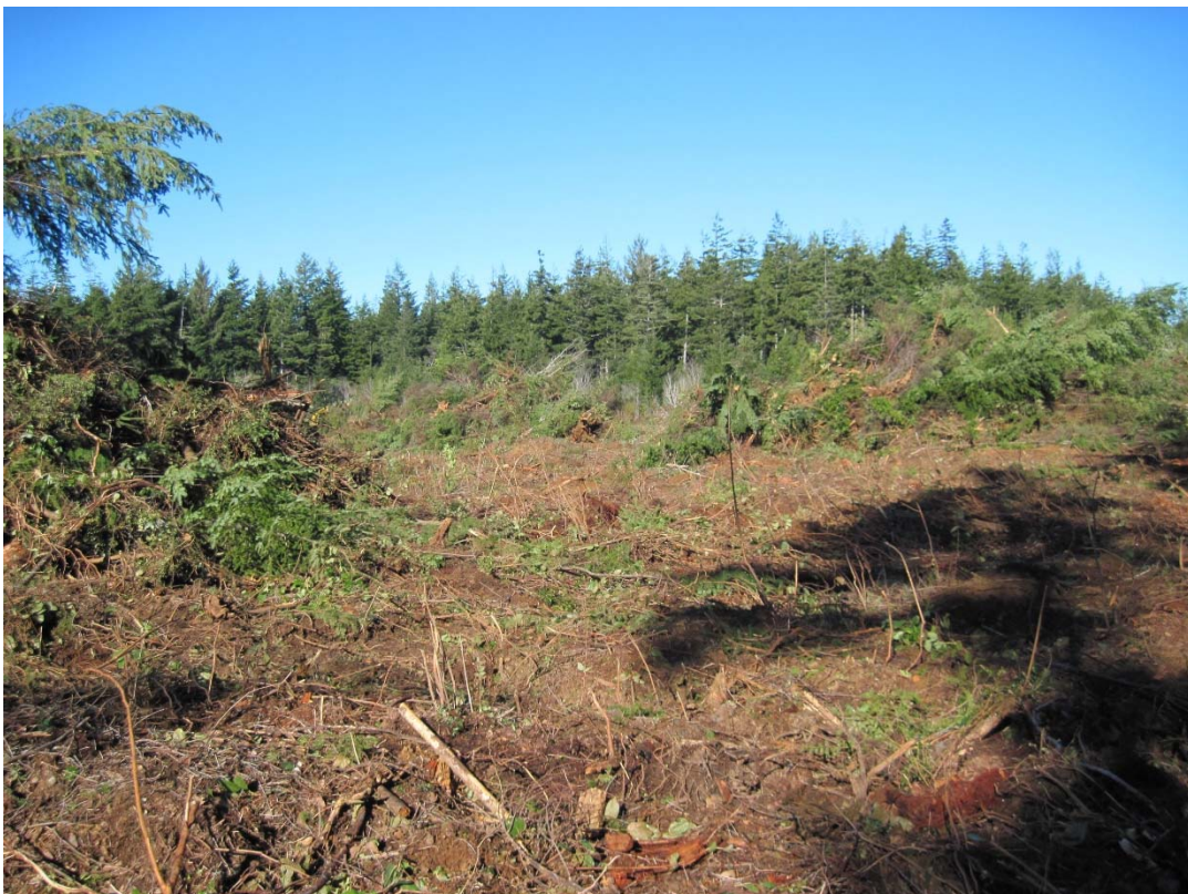
Photo 4. View of site after brush clearing
