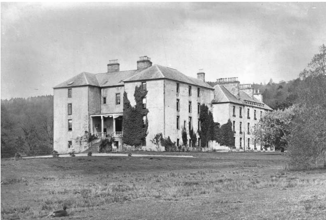
Brahan before demolition
