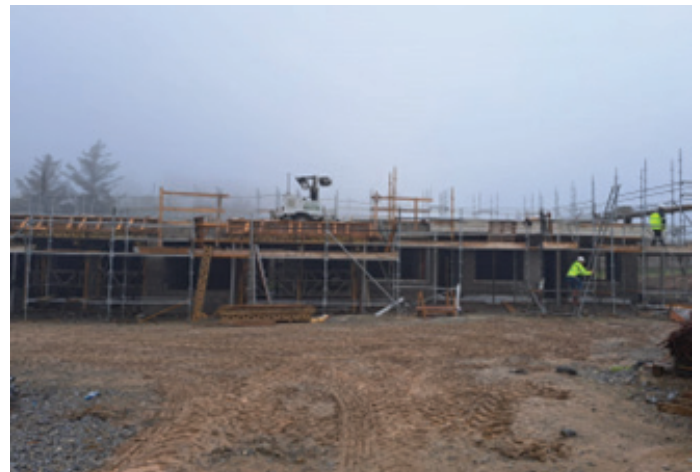
Progress on Scarriff housing development
