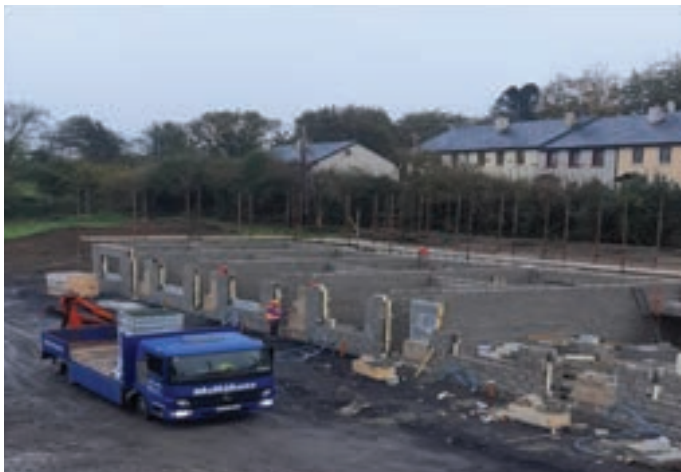
Works ongoing on Sixmilebridge project
