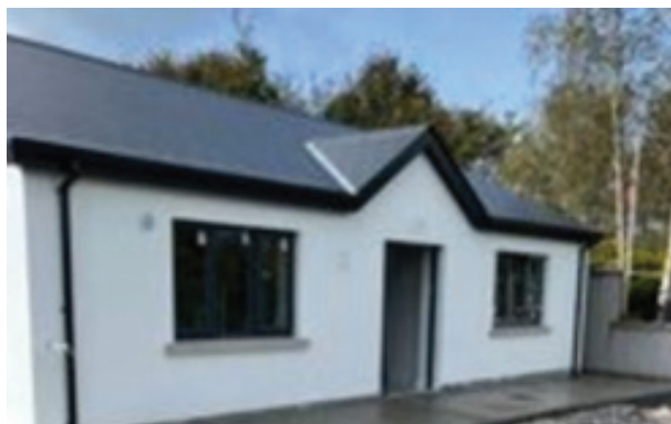
Works progressing on Clarecastle project
