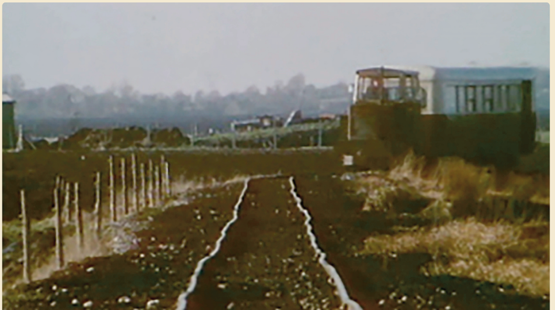
Fig 4: Derrygreenagh Bog Rail Network, RTE Archive
