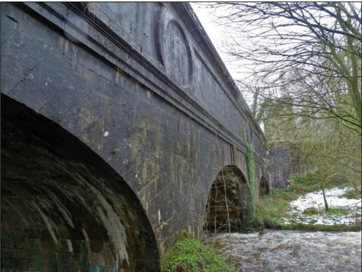
Dukart's aqueduct, Newmills.
