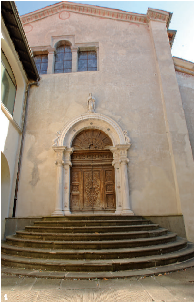
1 Stairs and access portal to Pieve
