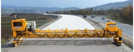
Texture/cure machine (GOMACO T/C-600 ). Follows the paver applying a white curing compound
