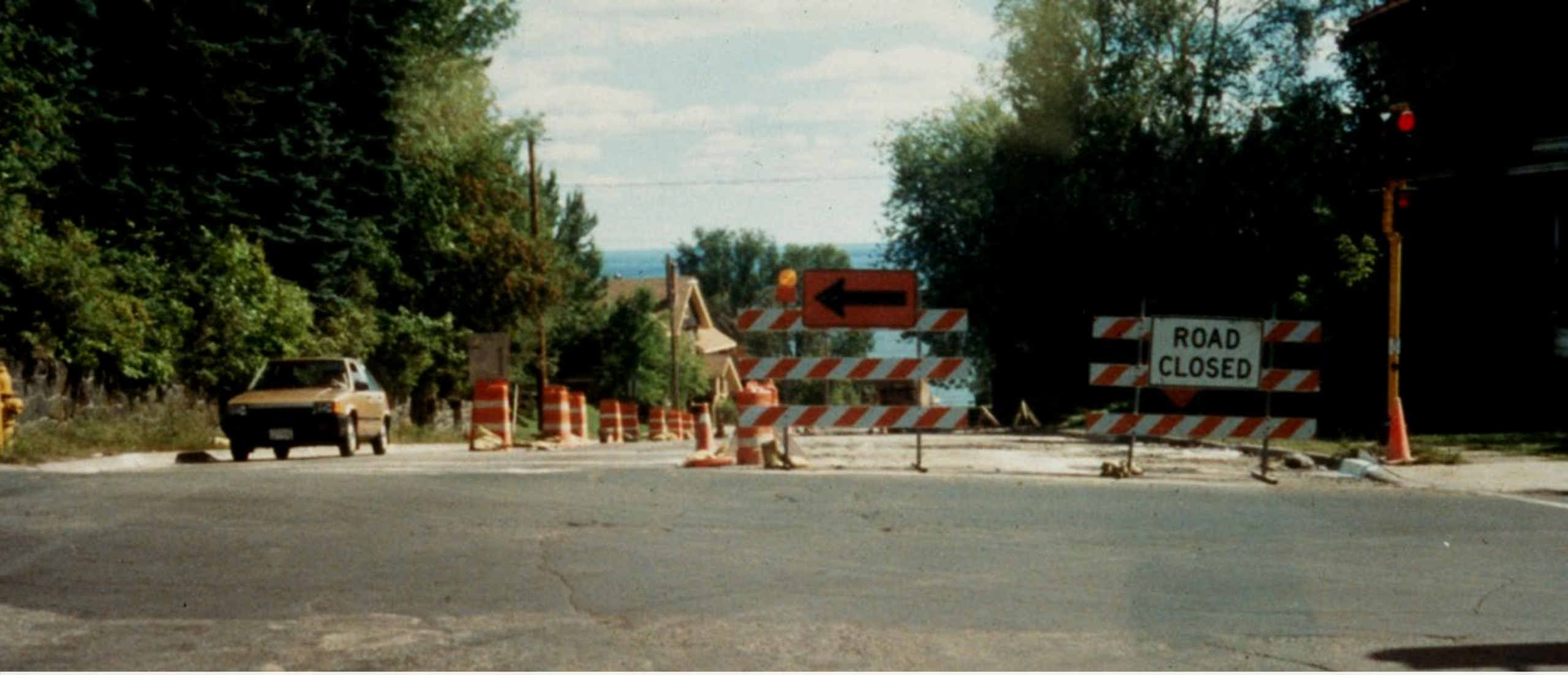
Roadway Closed with Marked Detour... Every other (staged) cross road closures
