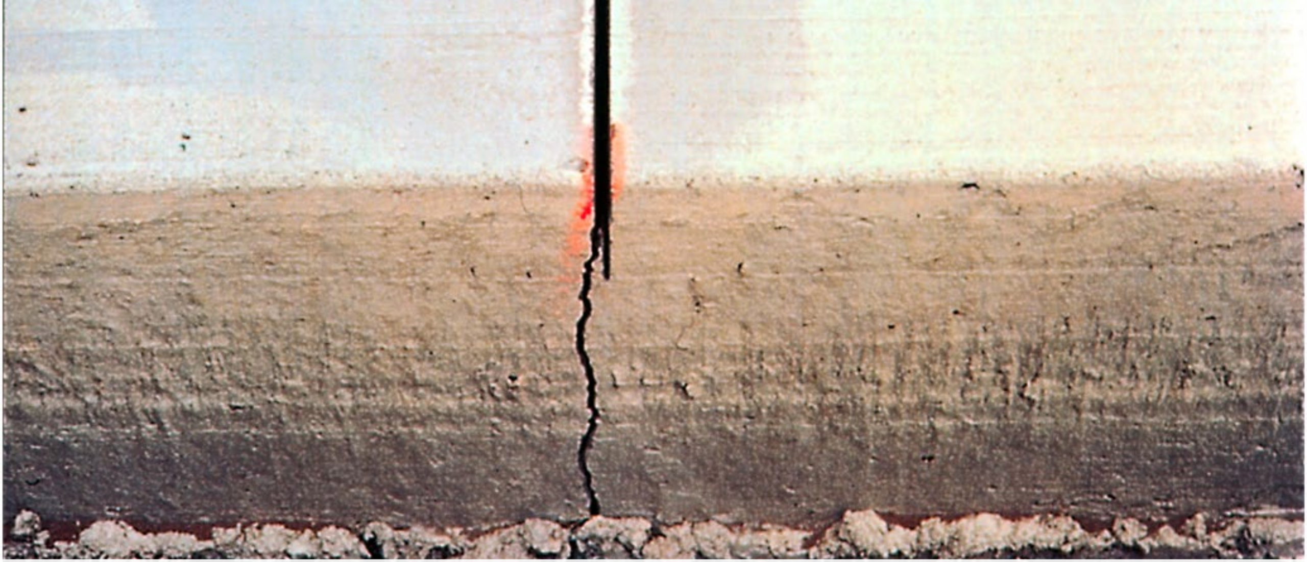
Transverse Contraction Joints
